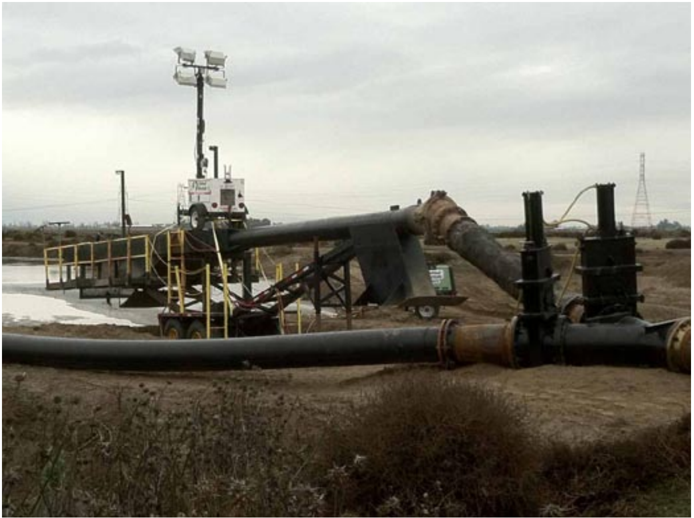
Figure 3. Photograph of discharge pipeline y-valve
