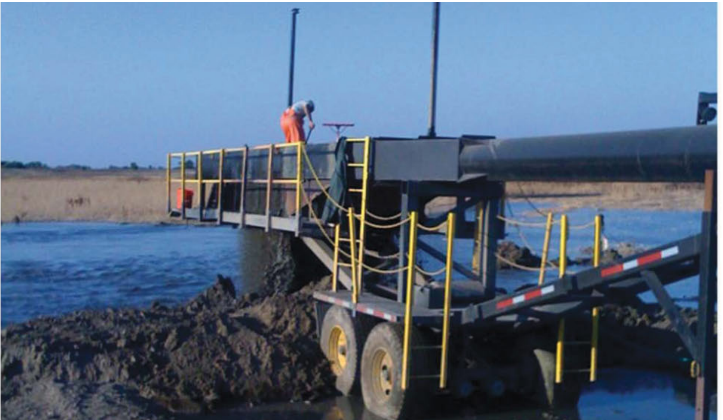
Figure 5. Entrapment Screen in Position and in Use at DMP Sites
